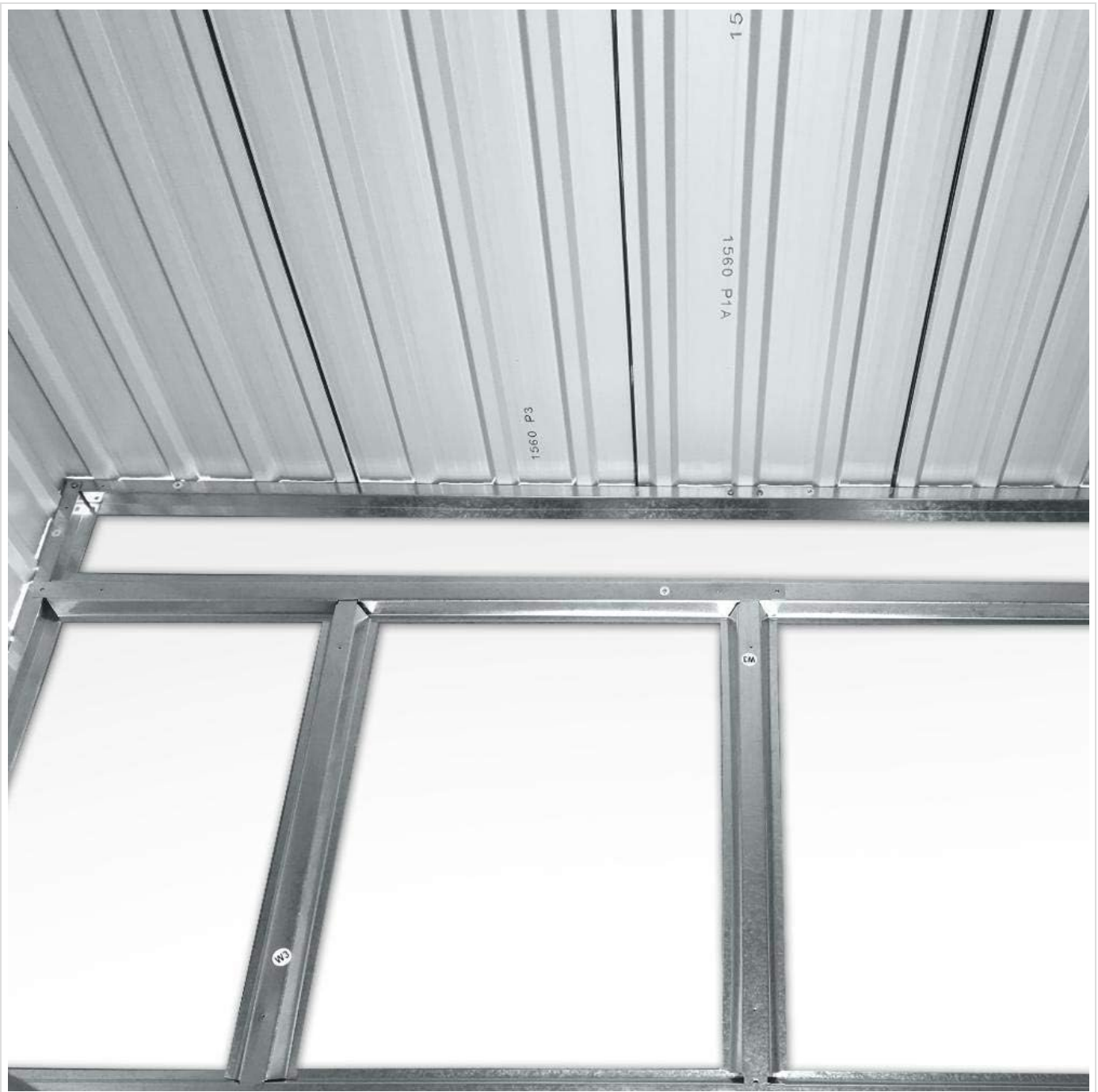
Figure 4: Interior Roof View. This perspective illustrates the internal structure of the roof and how panels are joined.
