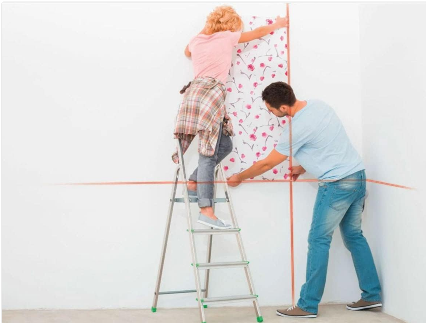
Figure 5: Example of the laser level being used in a practical application, assisting with wallpaper installation.
