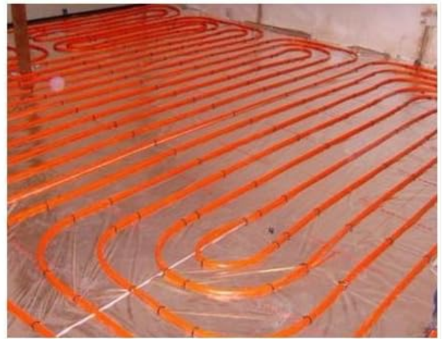
Wall-hung boiler heating
