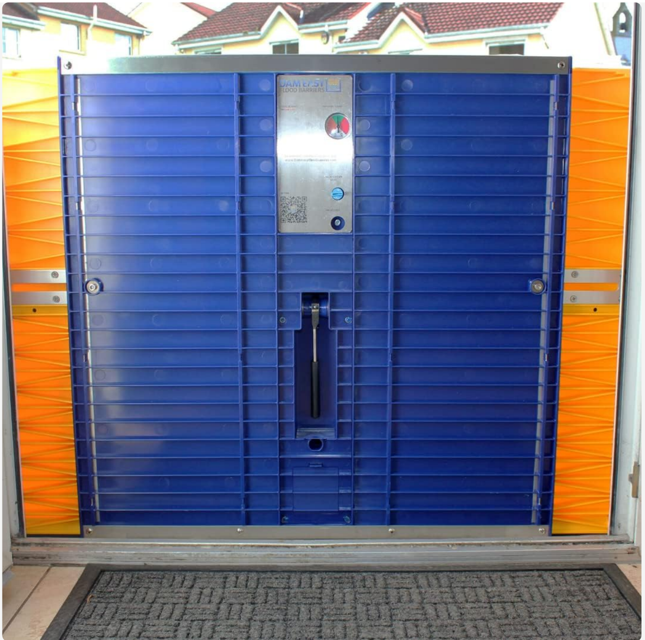
Figure 4.3: The Dam Easy Flood Barrier installed from the interior side of a doorway.
