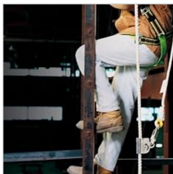
Image 3.1: Worker utilizing the harness during climbing activities, connected to a fall protection system.
