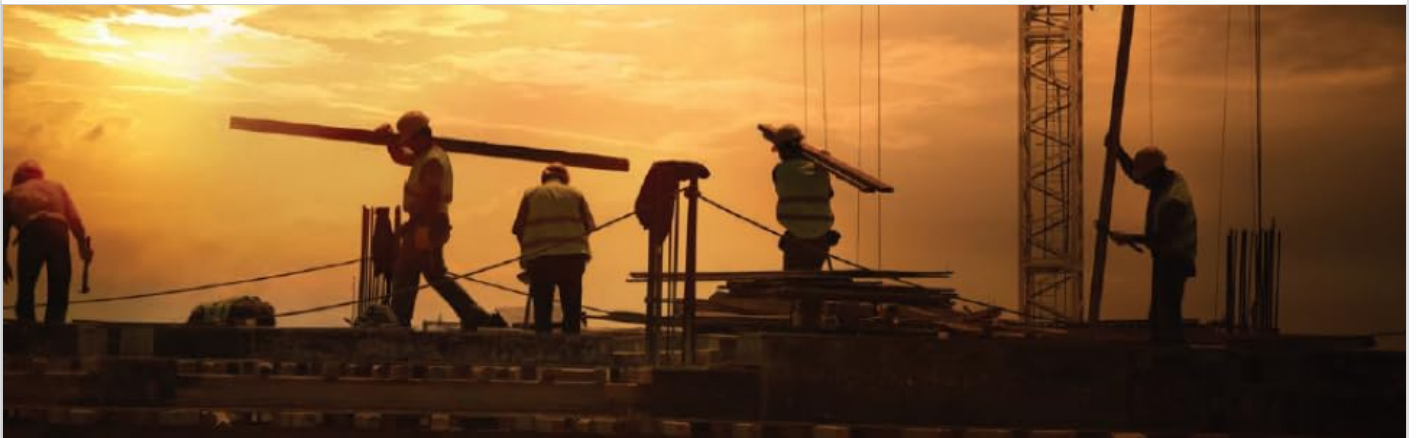
Image 0.1: General view of a construction site, highlighting the importance of safety equipment.
