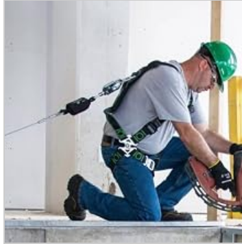
Image 2.2: Side view of a worker wearing the harness, demonstrating proper fit during activity.
