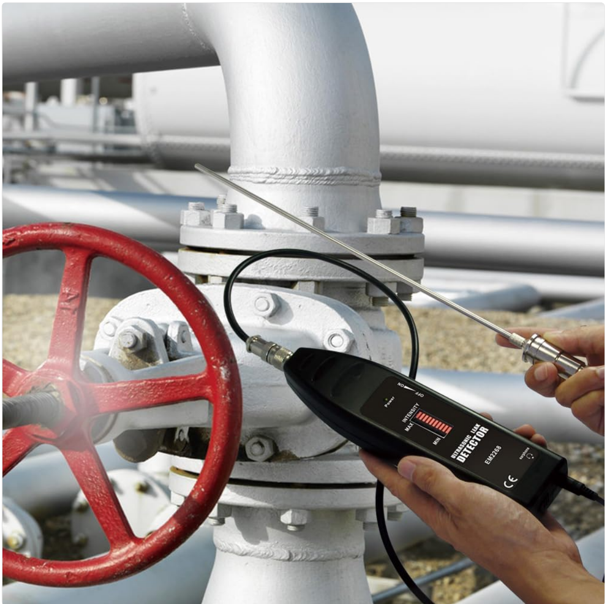
Figure 5: Using the contact probe for mechanical diagnosis on a pipe valve.
