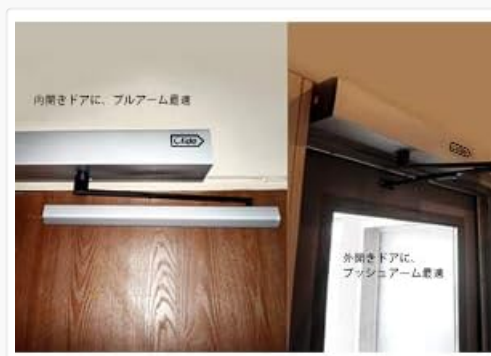
Figure 3.1: Illustration showing the optimal arm configuration for inward-opening doors (pull arm) and outward-opening doors (push arm).
