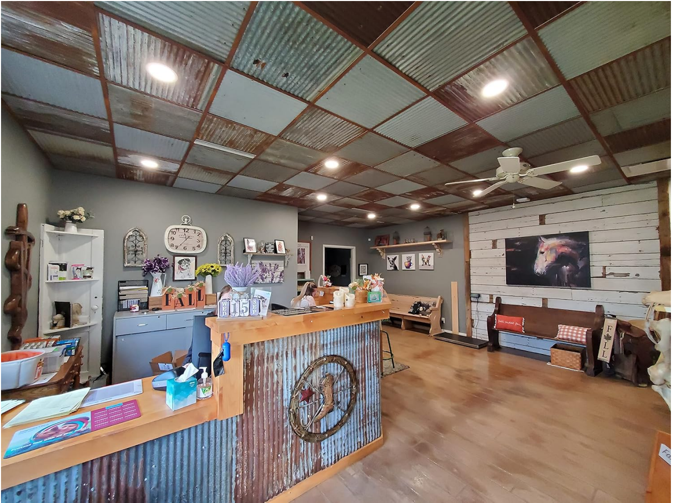
Figure 9.2: High ceiling application of mixed tin tiles with modern lighting.
