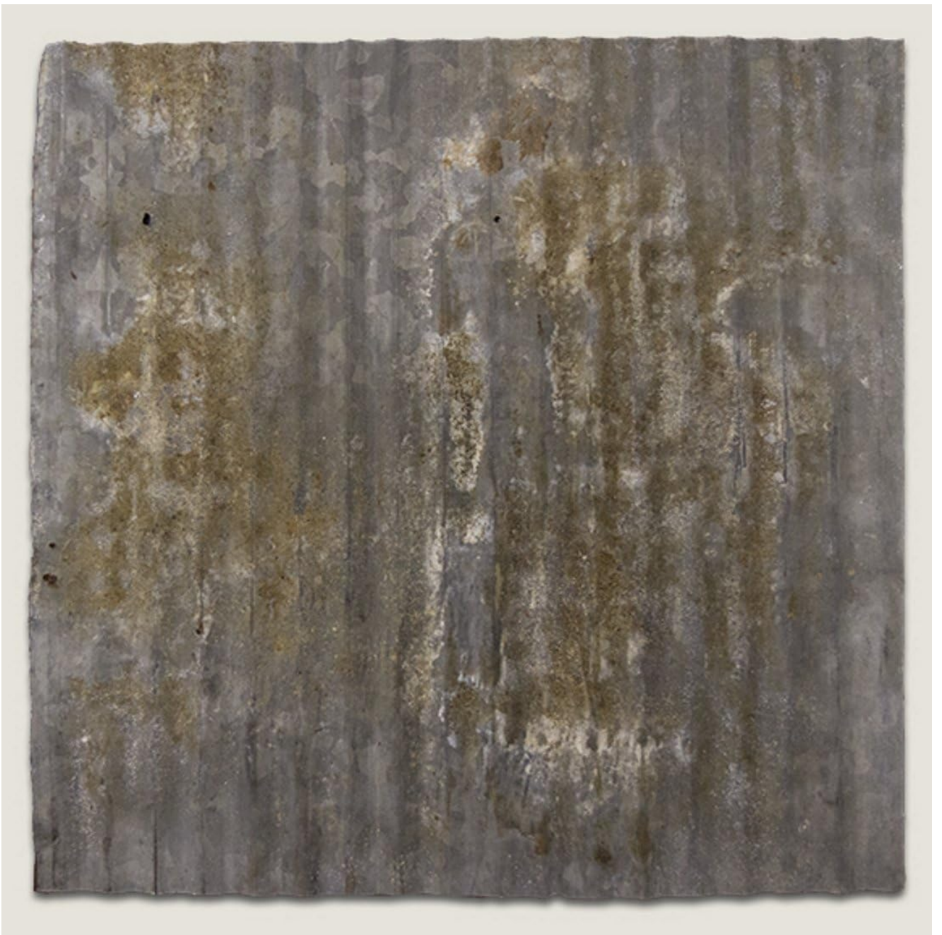
Figure 9.5: Detail of a galvanized corrugated tin tile.
