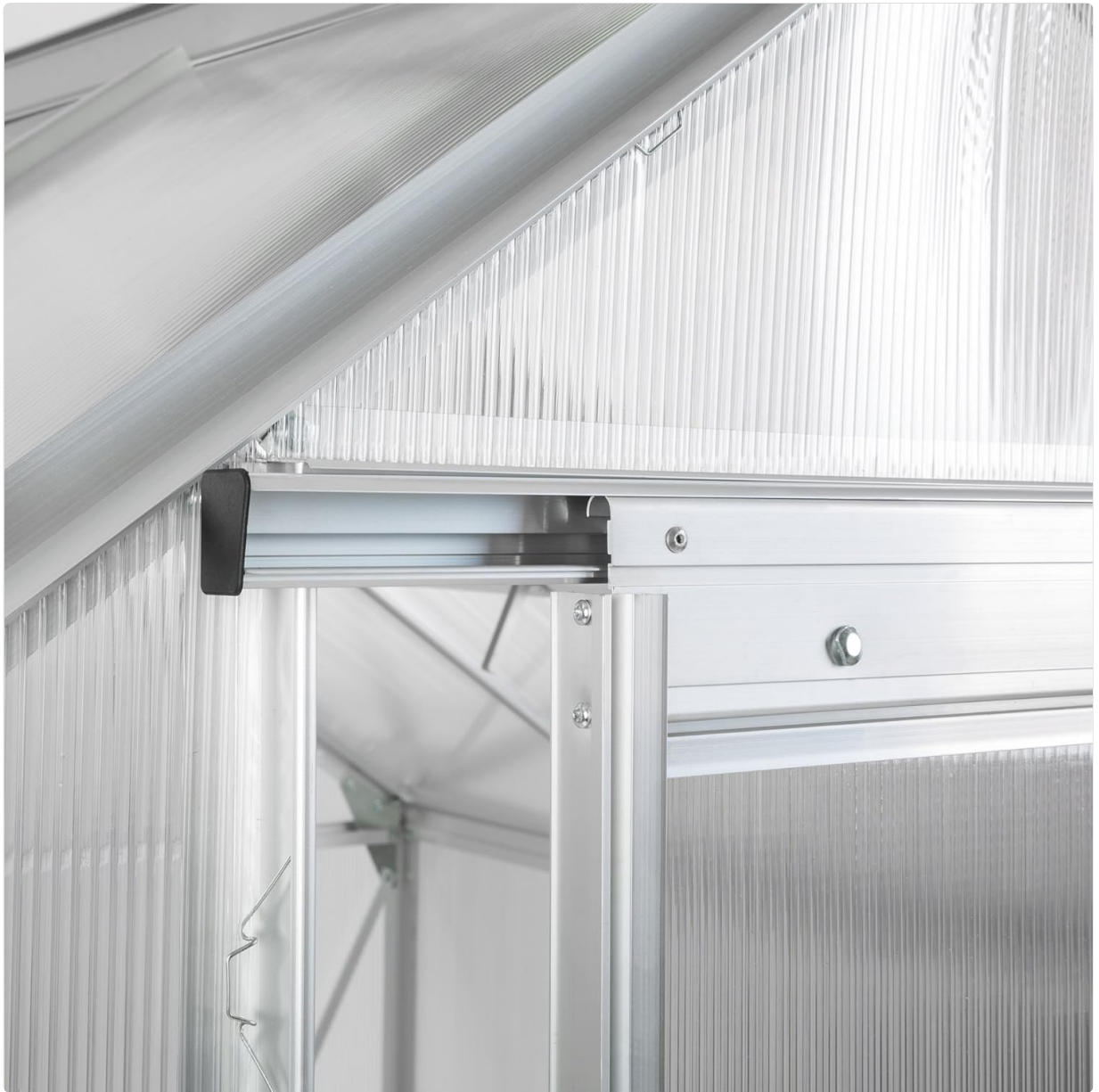
Image: A detailed shot of the sliding door's upper track and roller mechanism, indicating smooth operation.
