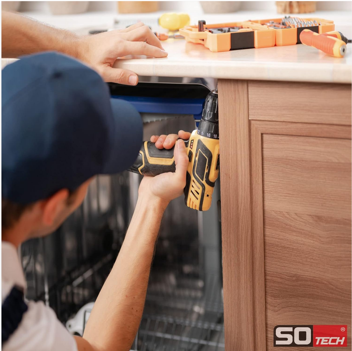
Figure 3: Installation in progress. This image shows a person actively installing the SOTECH steam protection plate. They are using a power drill to secure the plate to the underside of a kitchen countertop, directly above a built-in dishwasher.
