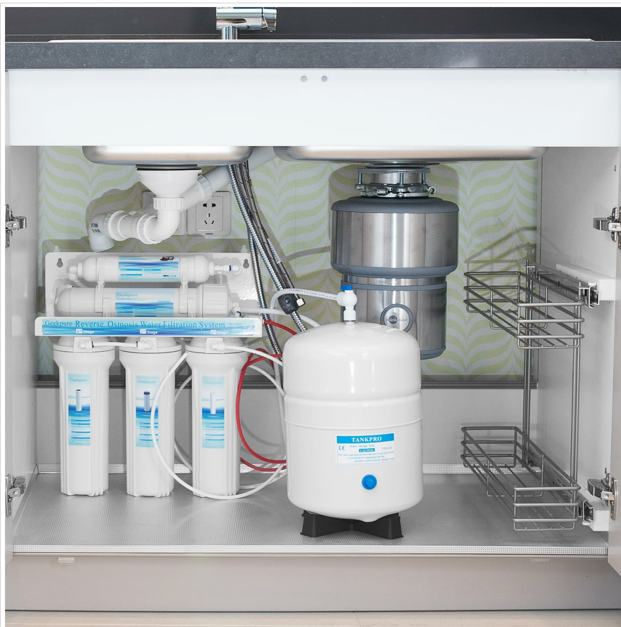
Figure 5: Example of under-sink installation.
