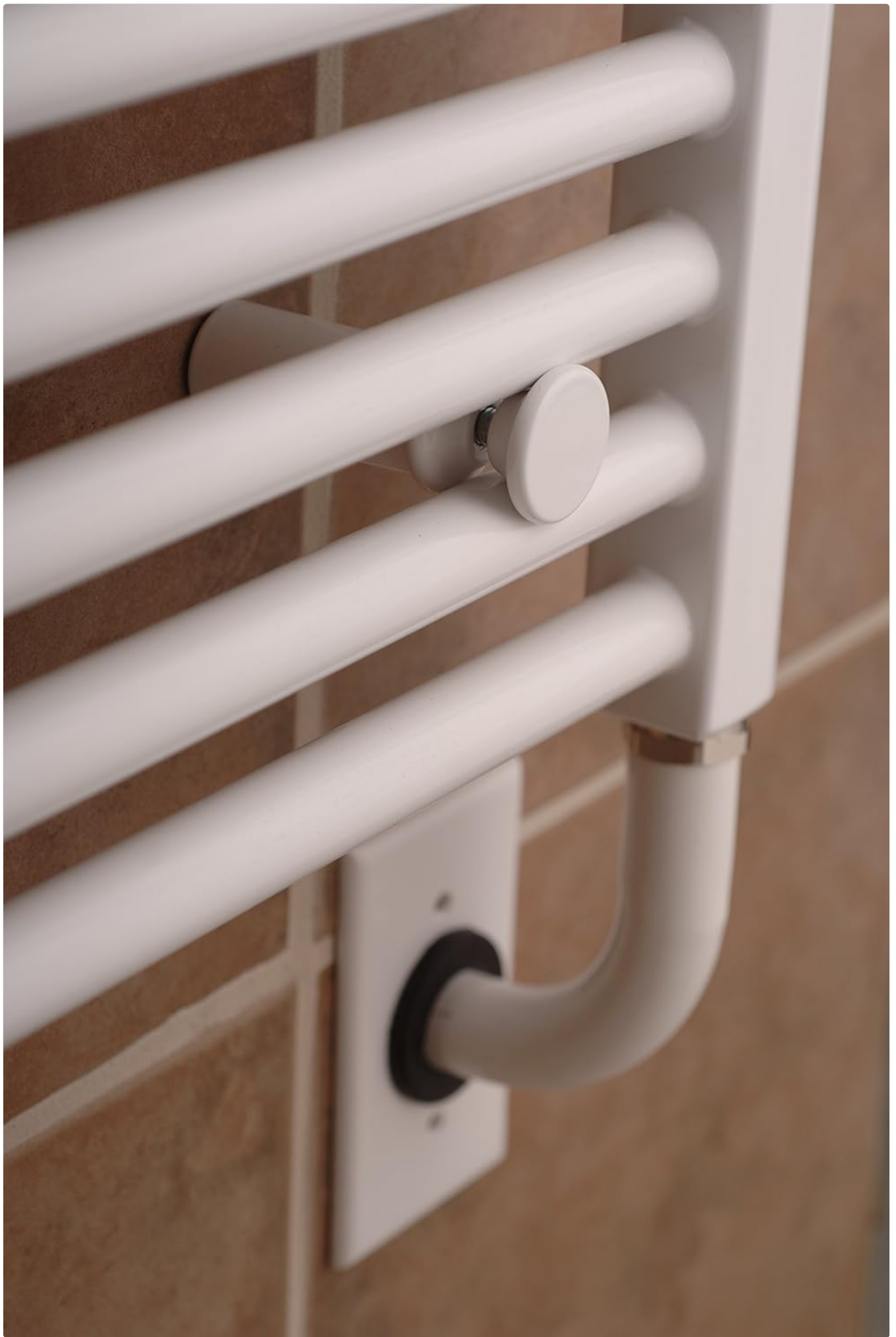
Image 3: Close-up view of the hardwire electrical connection point at the base of the towel warmer. This image details the conduit and
