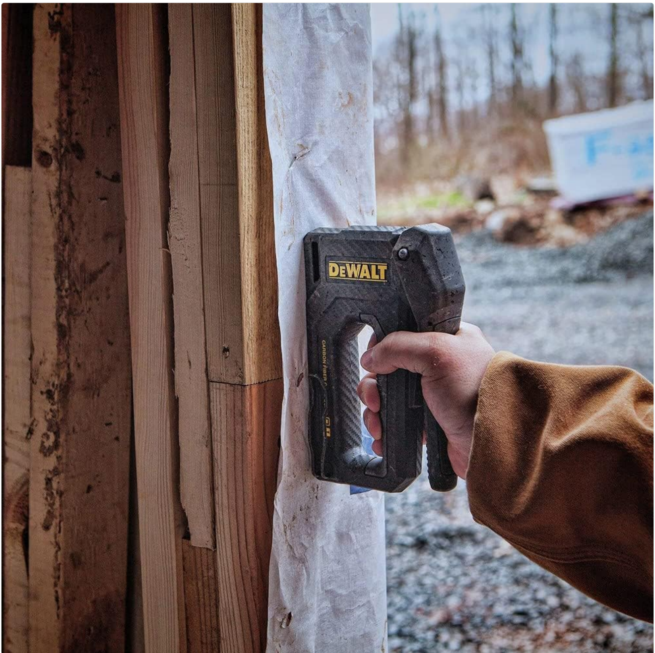
Image 5.1: Demonstrating the use of the tacker for securing insulation.
