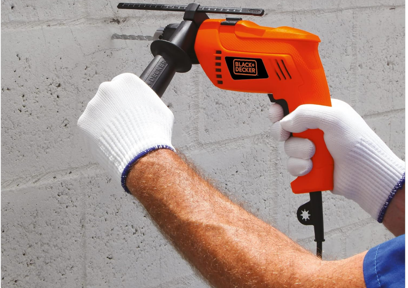
Figure 4: Drilling into concrete using the percussion mode.
