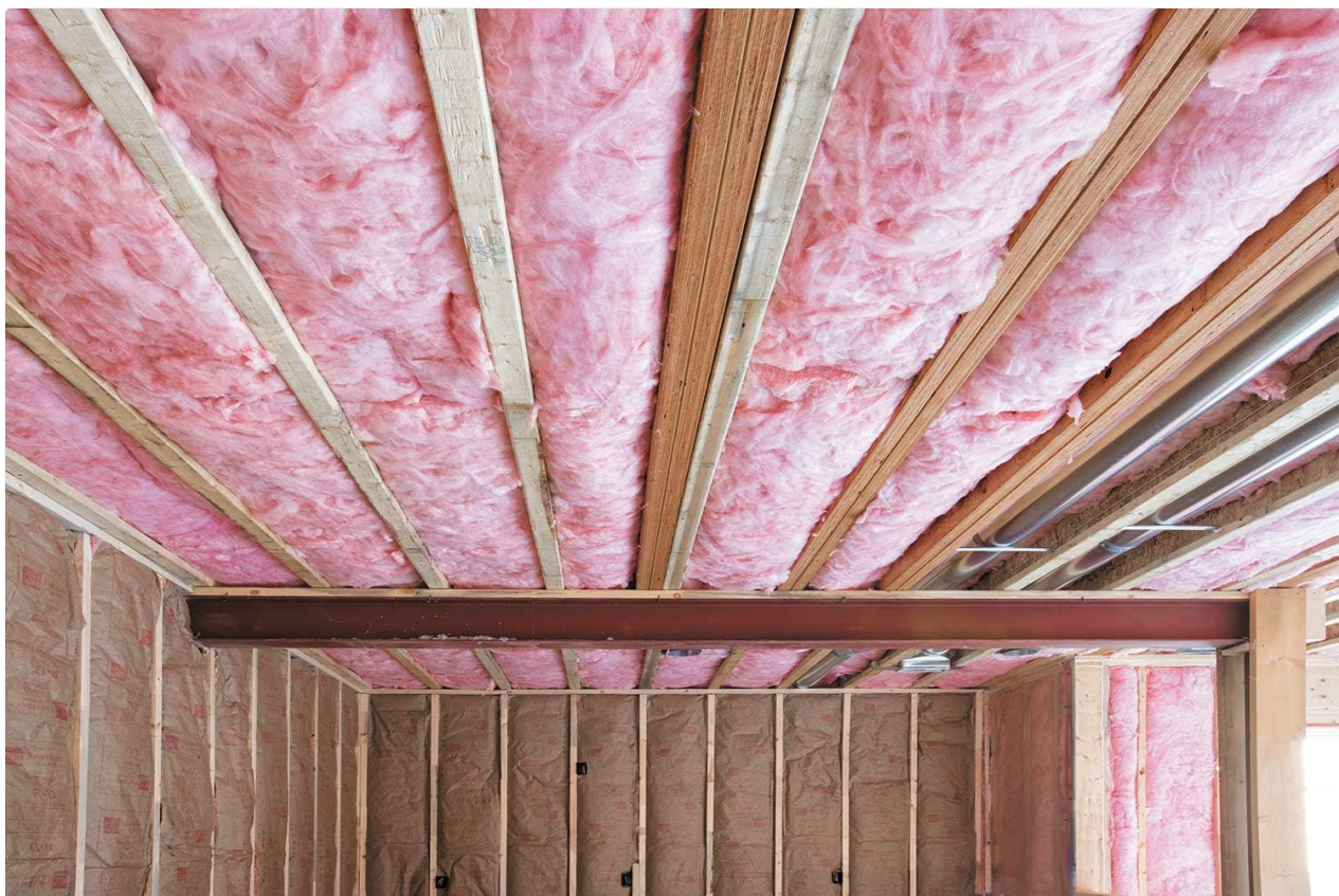
Figure 2.4: Owens Corning fiberglass insulation properly installed in a ceiling, filling the cavities.
