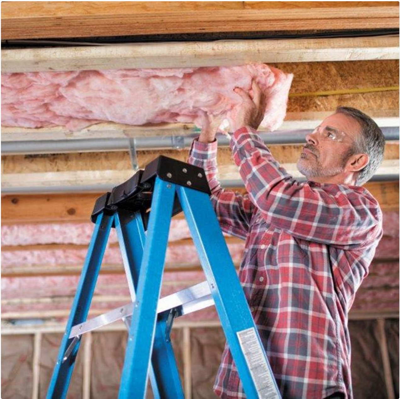
Figure 2.1: A man installing Owens Corning fiberglass insulation in a ceiling cavity.
