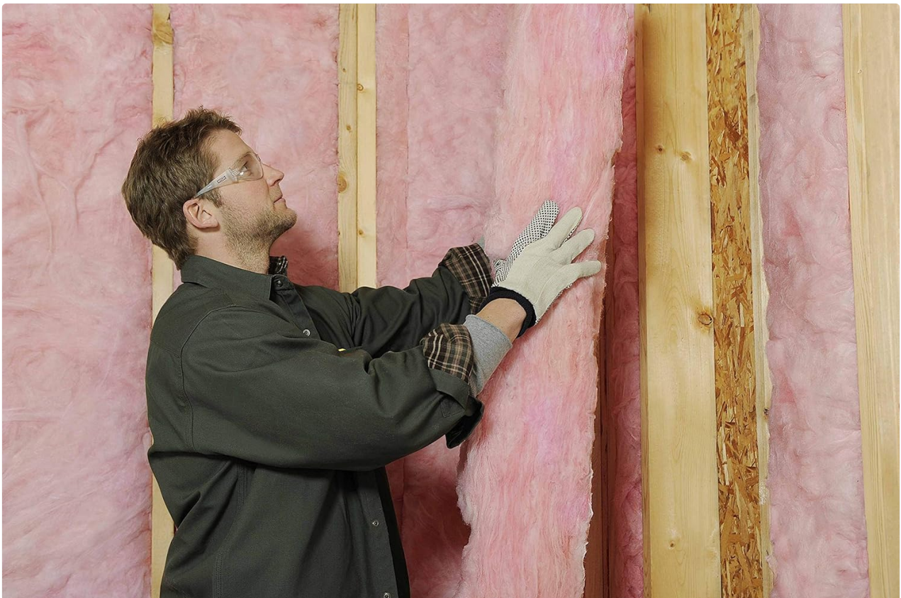
Figure 2.3: A man carefully fitting Owens Corning fiberglass insulation into a wall cavity.
