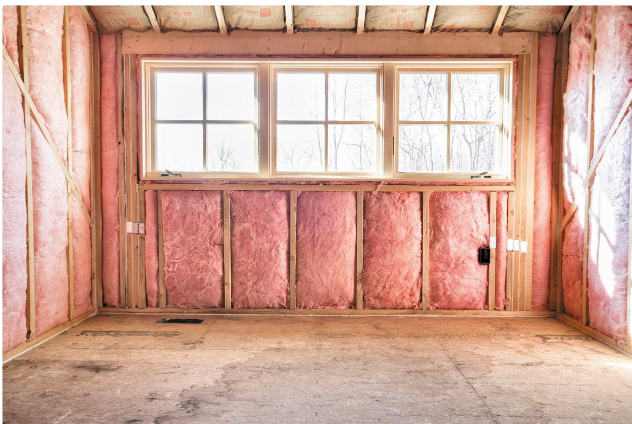
Figure 2.5: Owens Corning fiberglass insulation properly installed in wall cavities, including around a window opening.
