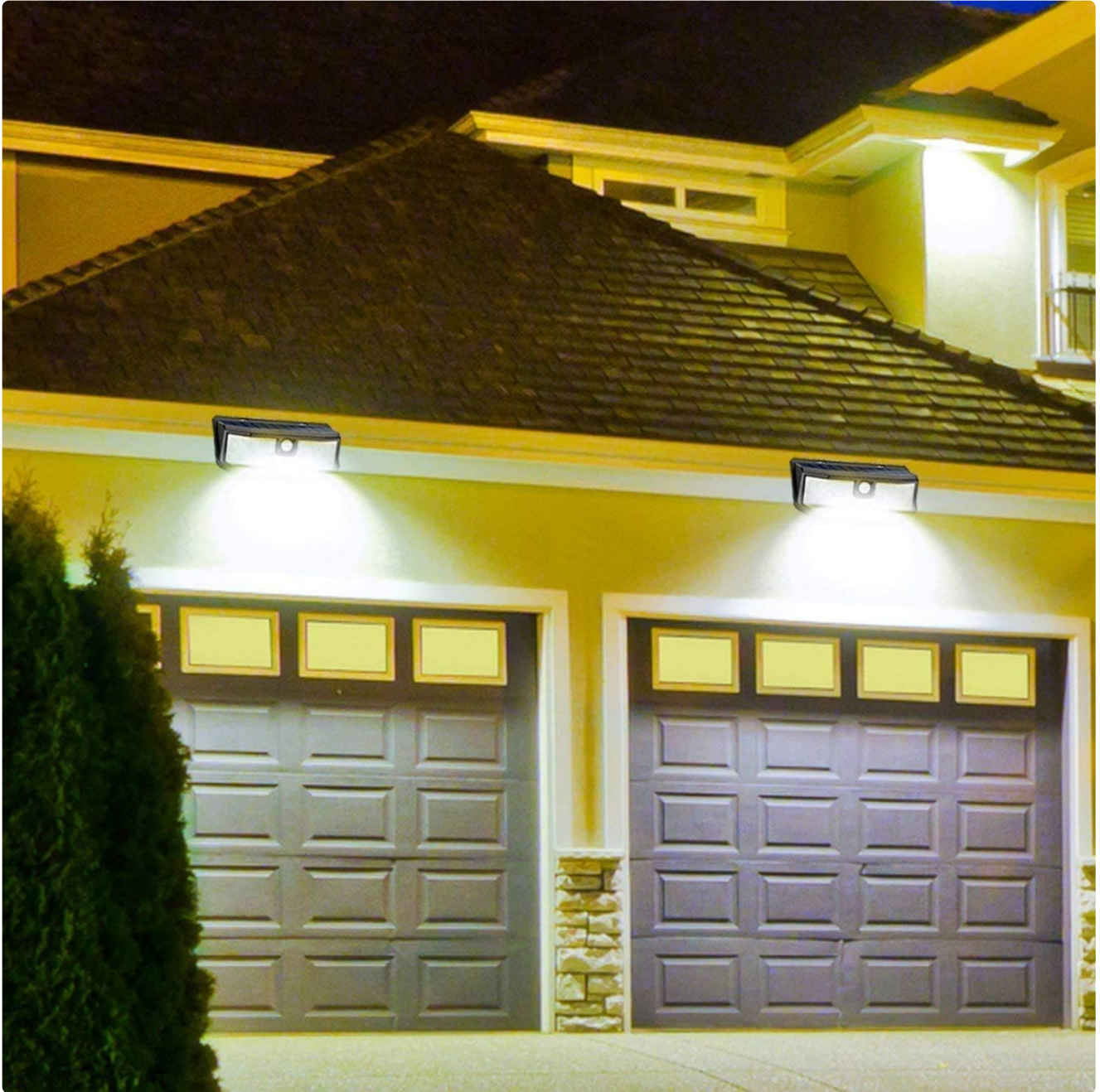
Figure 3.1: Example installation of Aootek Solar Lights above garage doors, demonstrating effective area lighting.
