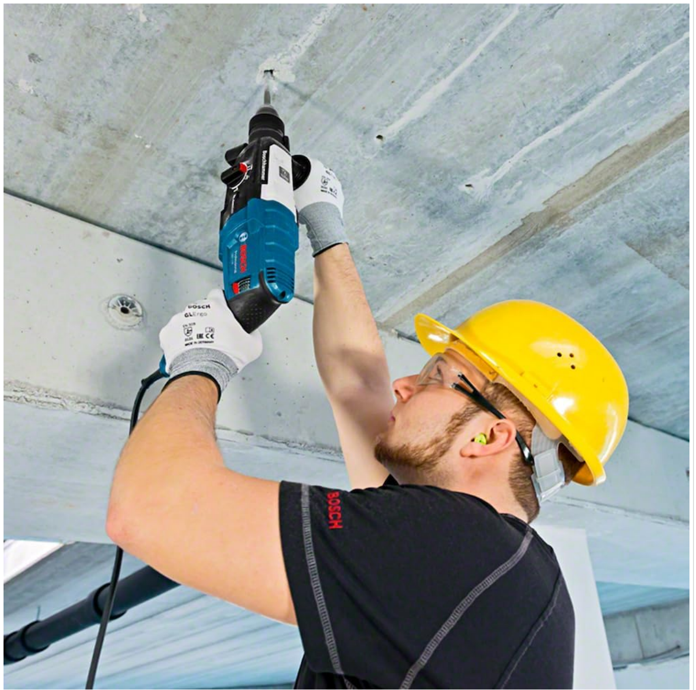
Figure 6: An individual performing overhead drilling into a concrete ceiling with the Bosch GBH 2-28D, wearing appropriate safety glasses, ear protection, and a hard hat.
