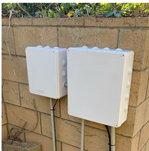
Figure 7: Multiple Box Installation Example
