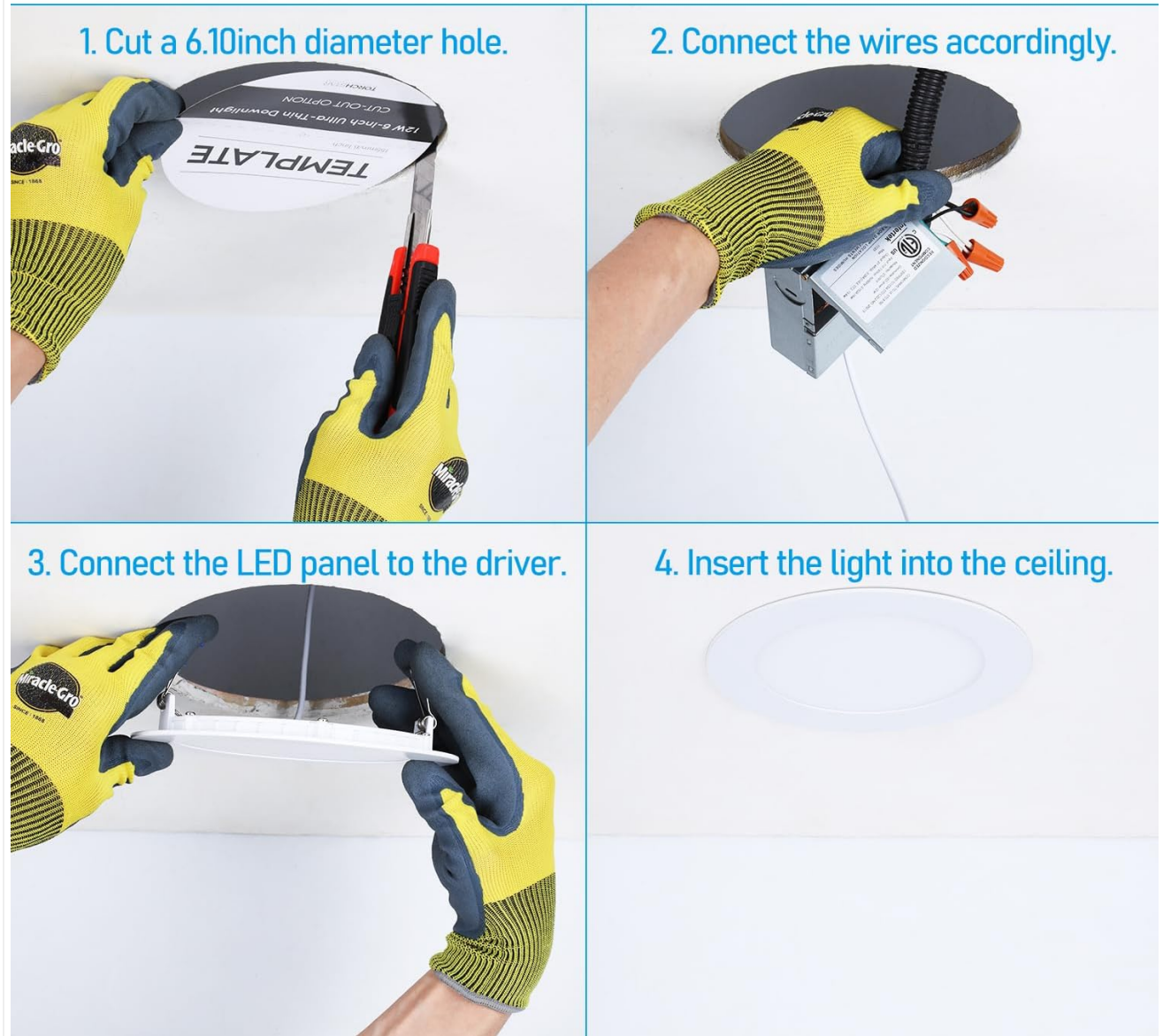
Image: Step 1 - Cutting a 6.10-inch diameter hole in the ceiling.
