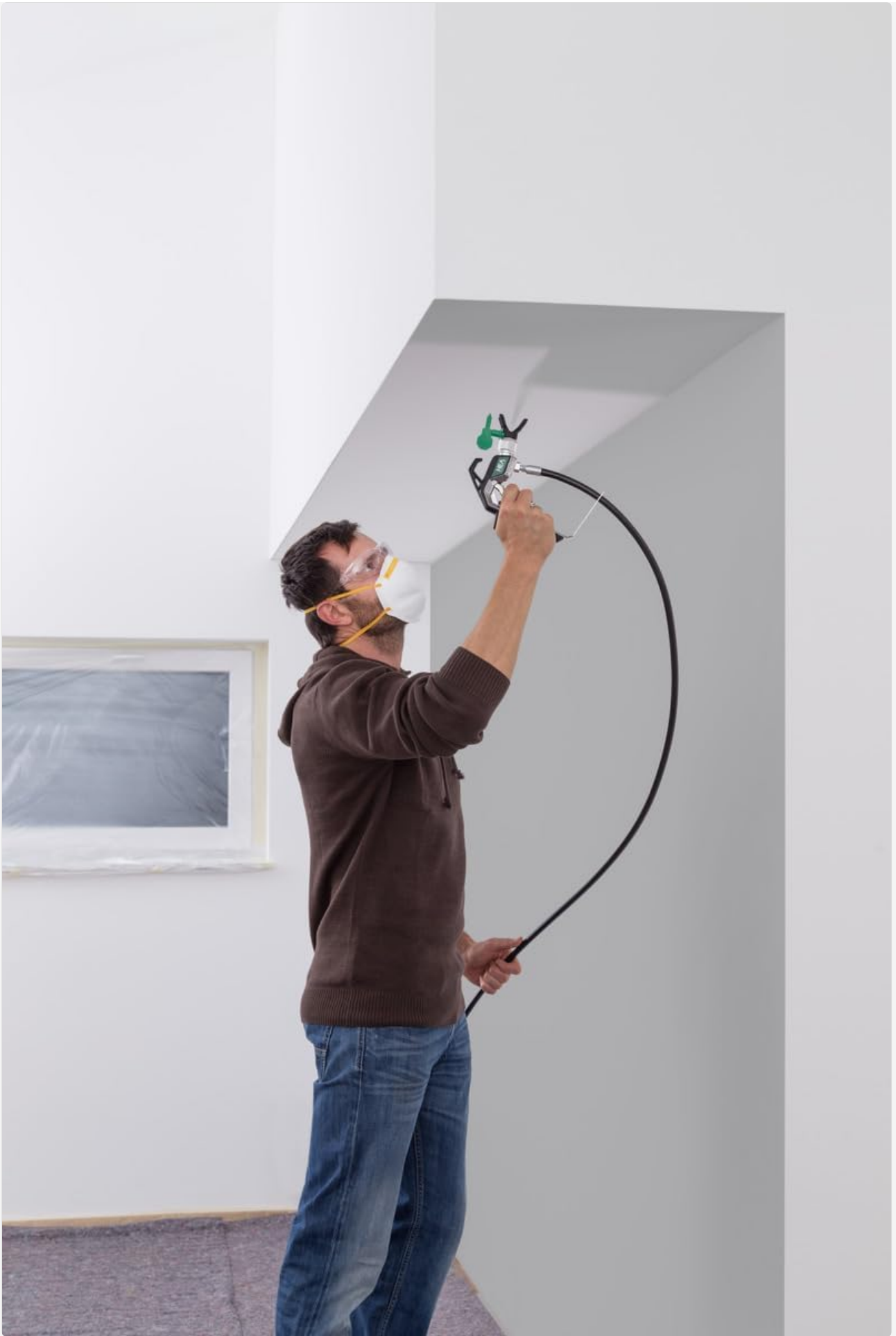
Image: An individual is shown spray painting an indoor ceiling with the WAGNER ControlPro 250R. The lightweight airless spray gun with its two-finger trigger allows for extended use without fatigue, making it suitable for overhead tasks.
