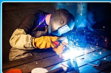
WELDING ANGLE IRON
