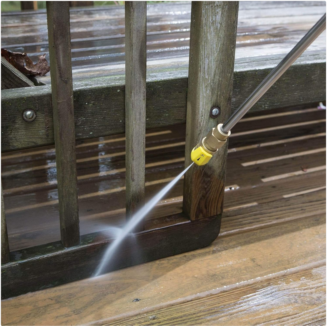
Figure 7: Applying detergent to a wooden deck for enhanced cleaning.
