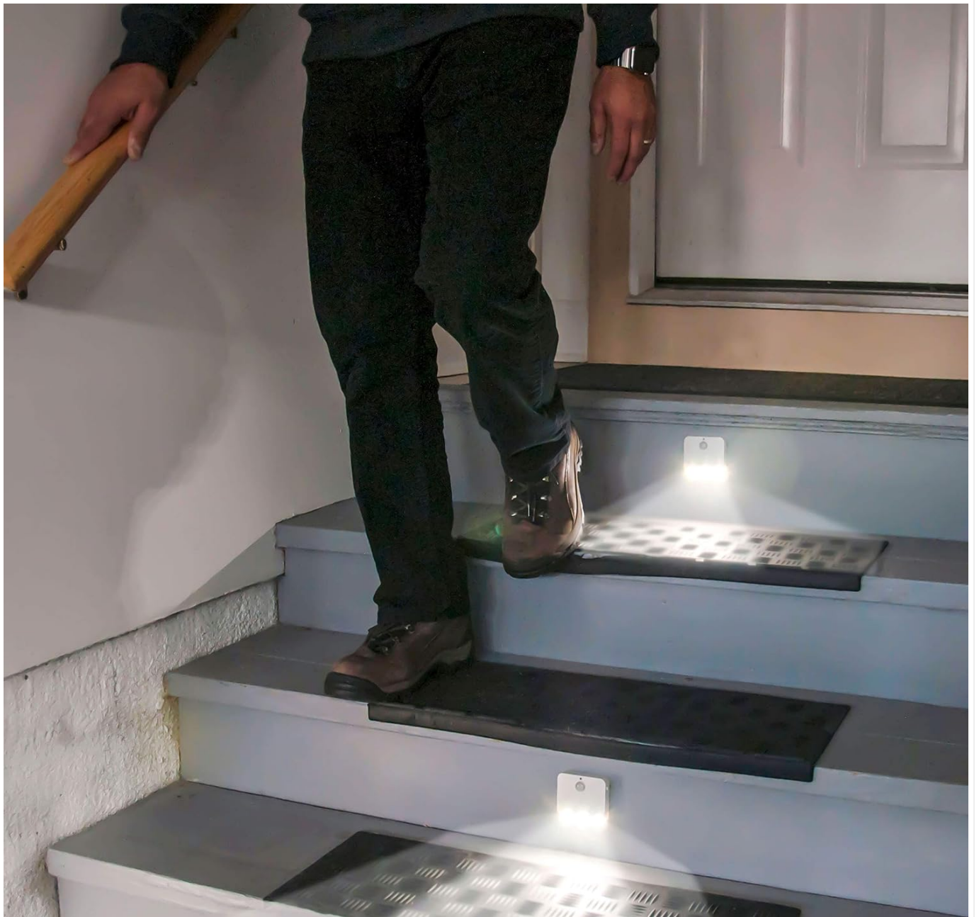
Image: Sensor Brite lights installed along a staircase, providing clear illumination for safe passage in the dark.
