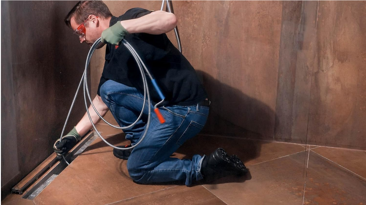
This image shows the user actively operating the drain cleaning spiral, demonstrating the technique of rotating the hand crank while guiding the spiral into the drain to clear a blockage.
