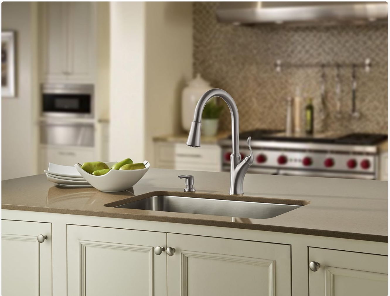
Image: The Pfister Eagan Faucet elegantly installed in a kitchen setting, demonstrating its functional design.
