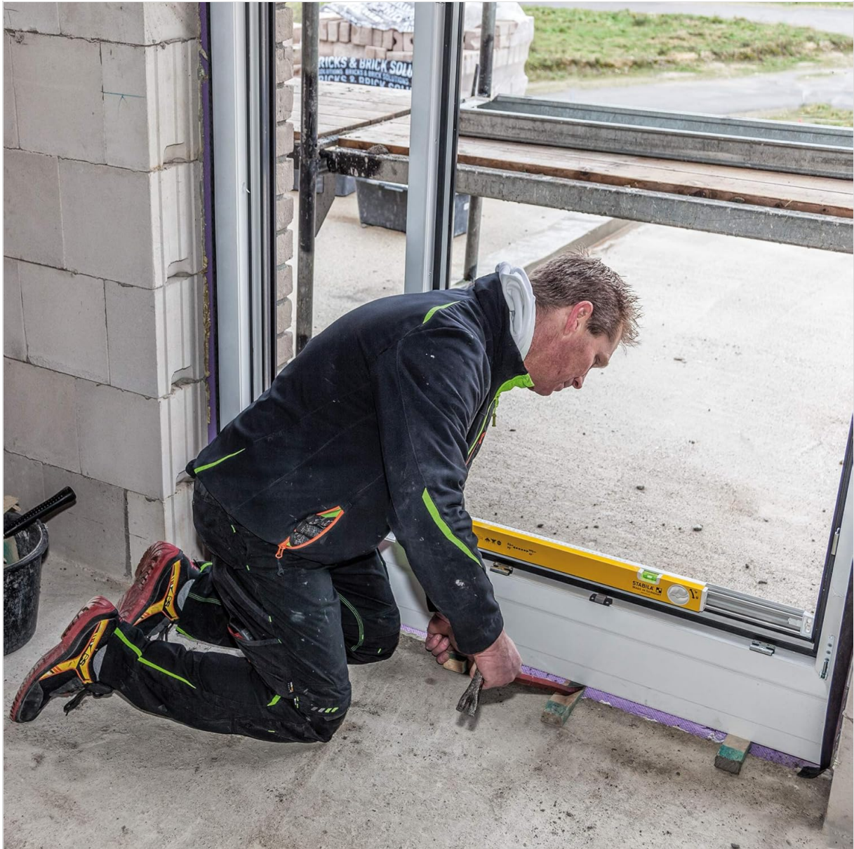
Image 4: A worker using the Stabila extendable level to check the horizontal alignment of a window frame during installation.
