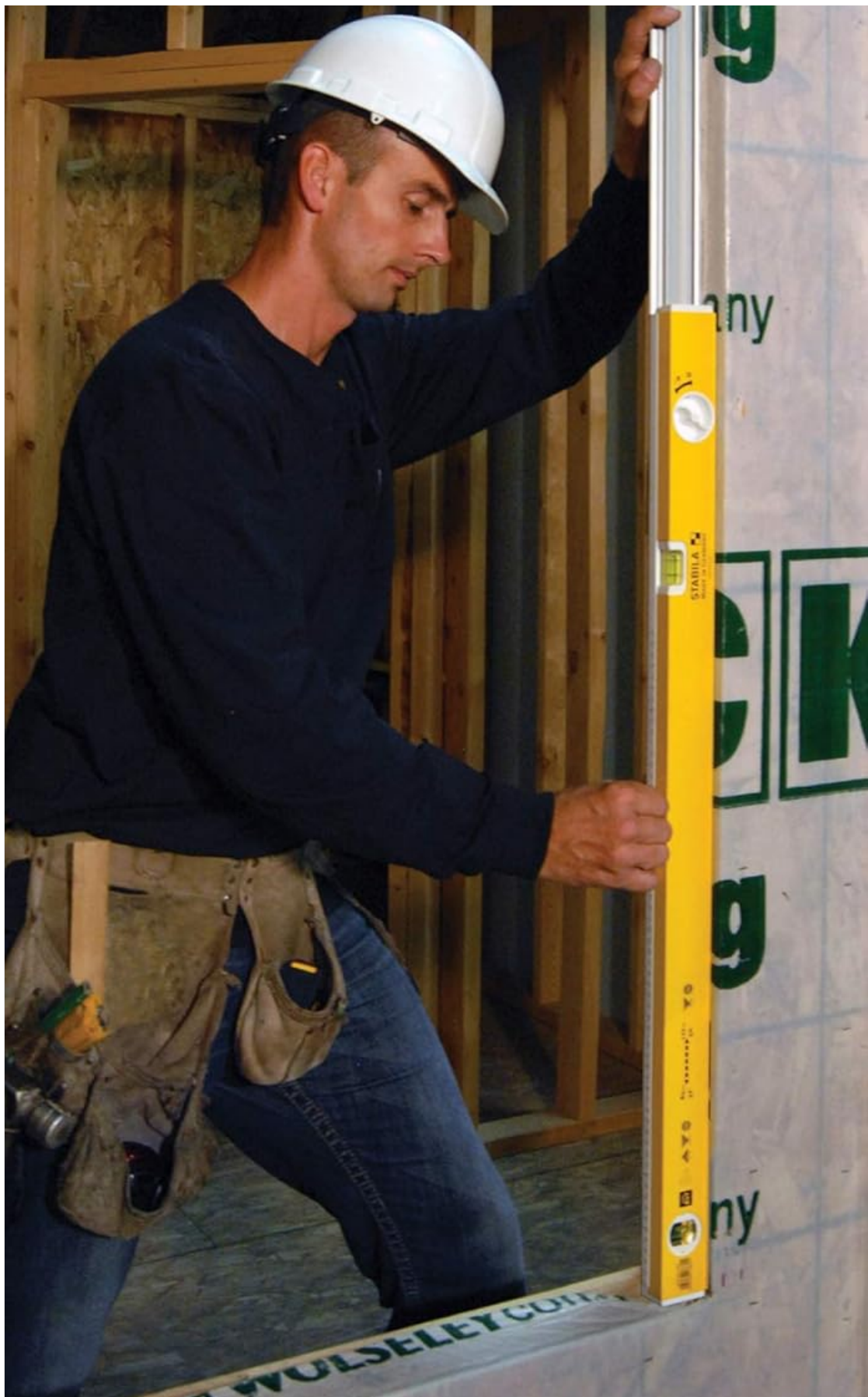
Image 5: A worker using the Stabila extendable level to verify the vertical alignment of a door frame, demonstrating its utility for tall structures.
