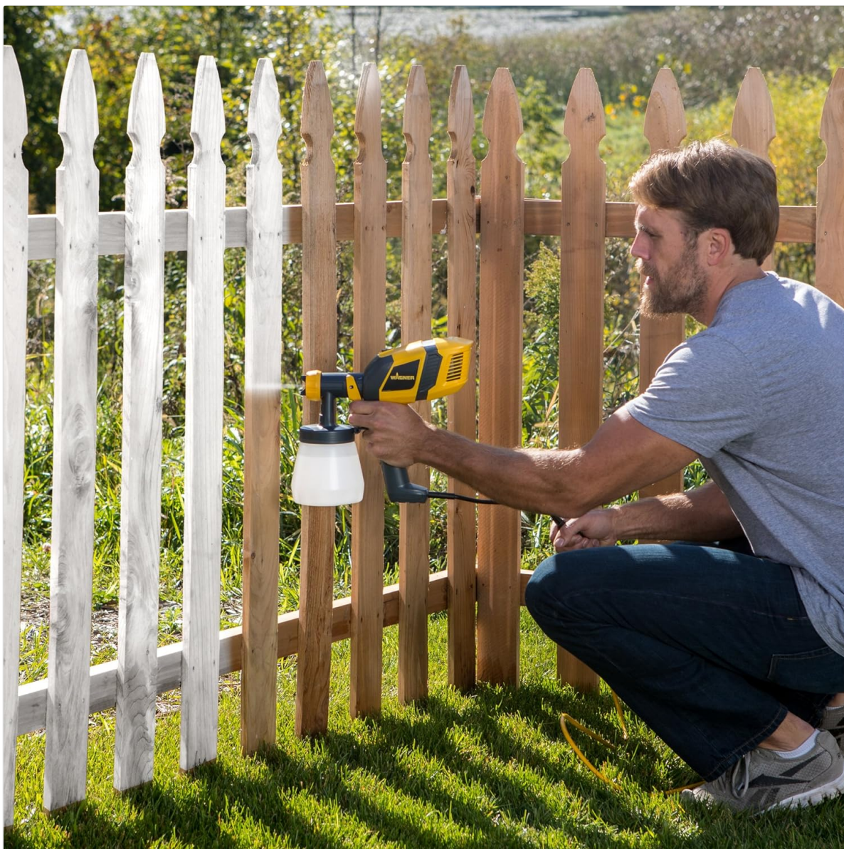
Image 5.1: A user demonstrating proper spraying technique on a picket fence, applying an even coat of material.
