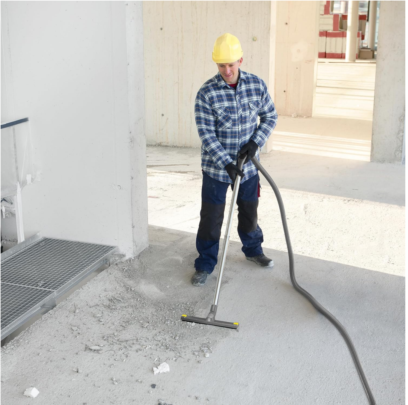
Figure 3: Operator using the Kärcher NT 30/1 Tact L to vacuum dry debris, demonstrating its effectiveness on construction sites or similar environments.
