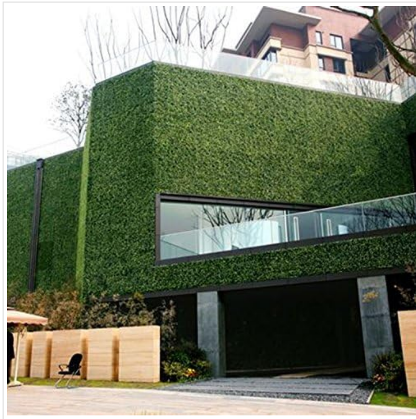
Figure 4: Large-scale application of artificial boxwood panels on a building exterior.
