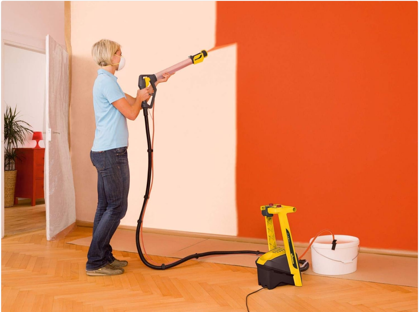
Figure 3: Applying paint to a wall using the spray lance.
