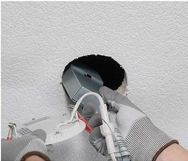
Figure 3: Ceiling Hole Preparation and Wiring
