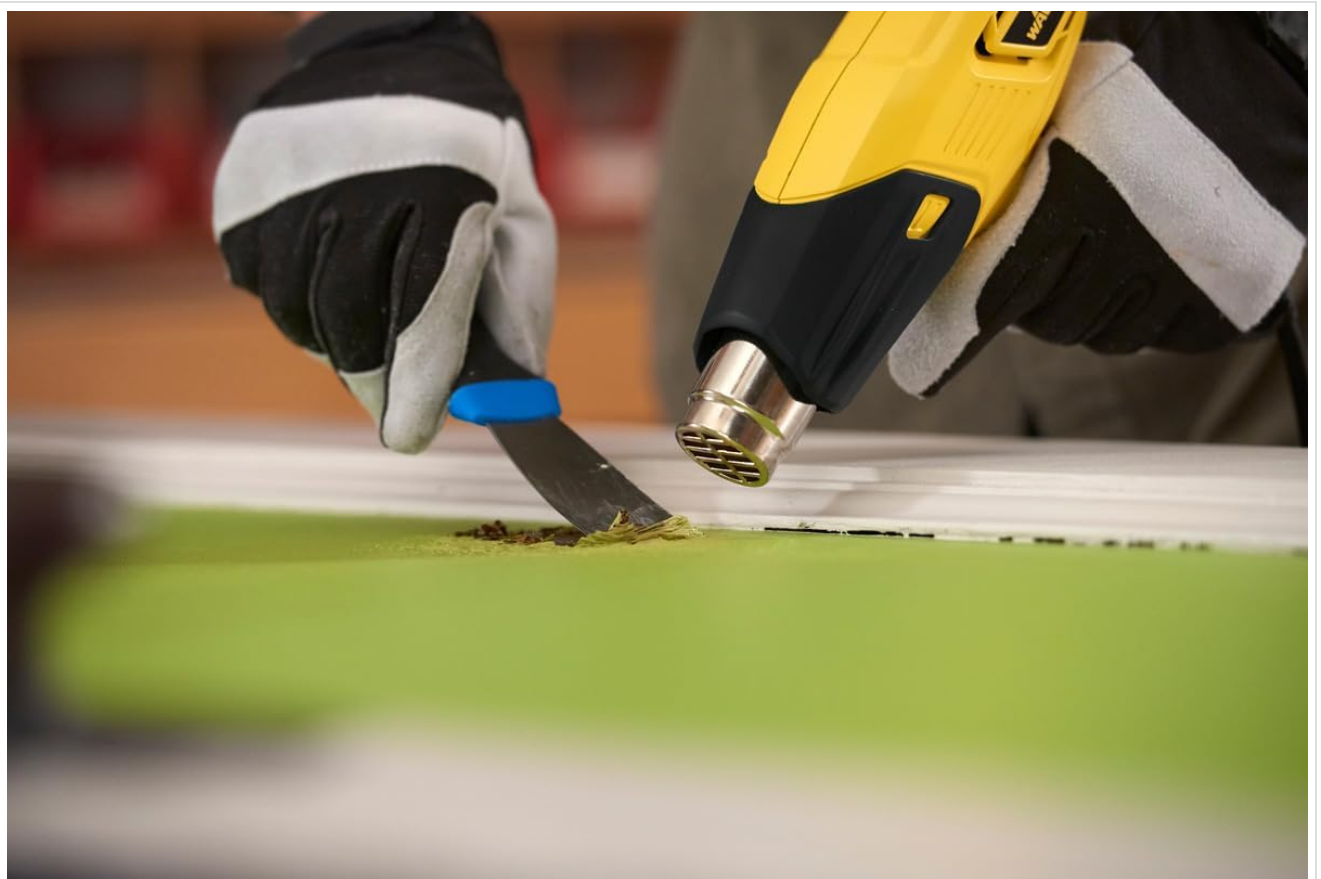
Figure 2: Using the heat gun for efficient paint removal from a surface.
