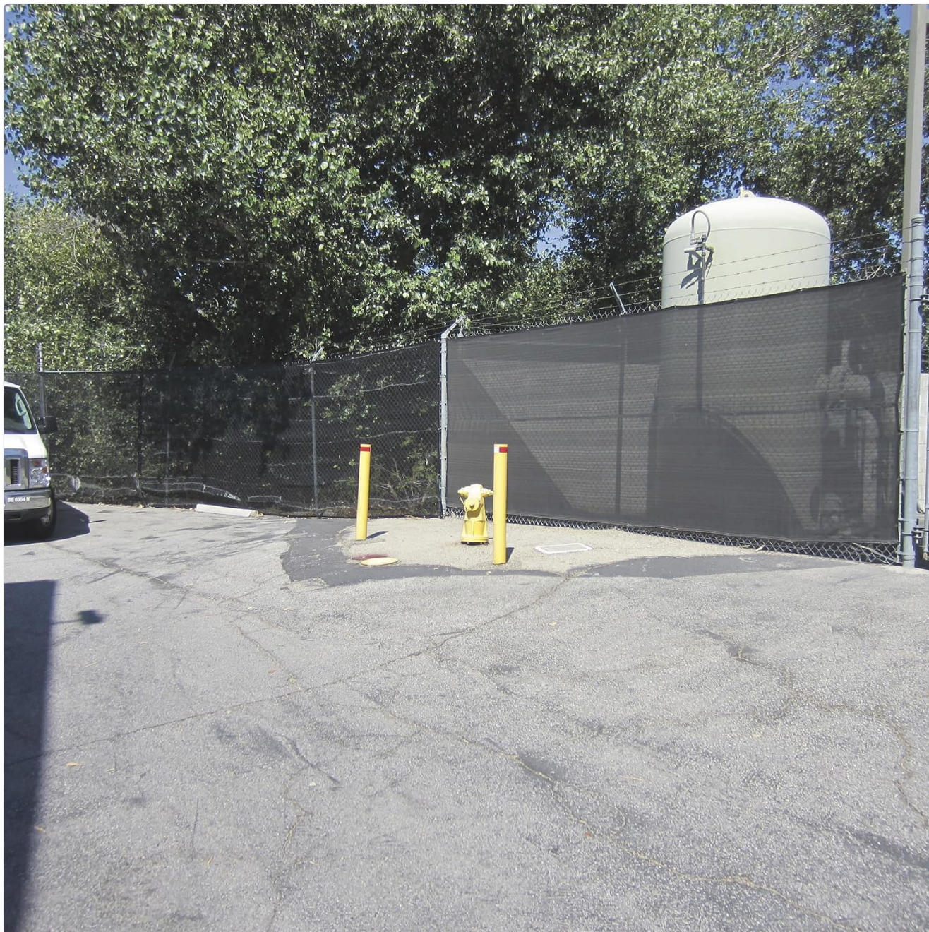
Image 2: Shade cloth installed along a chain-link fence, demonstrating its use as a privacy screen or windbreak.
