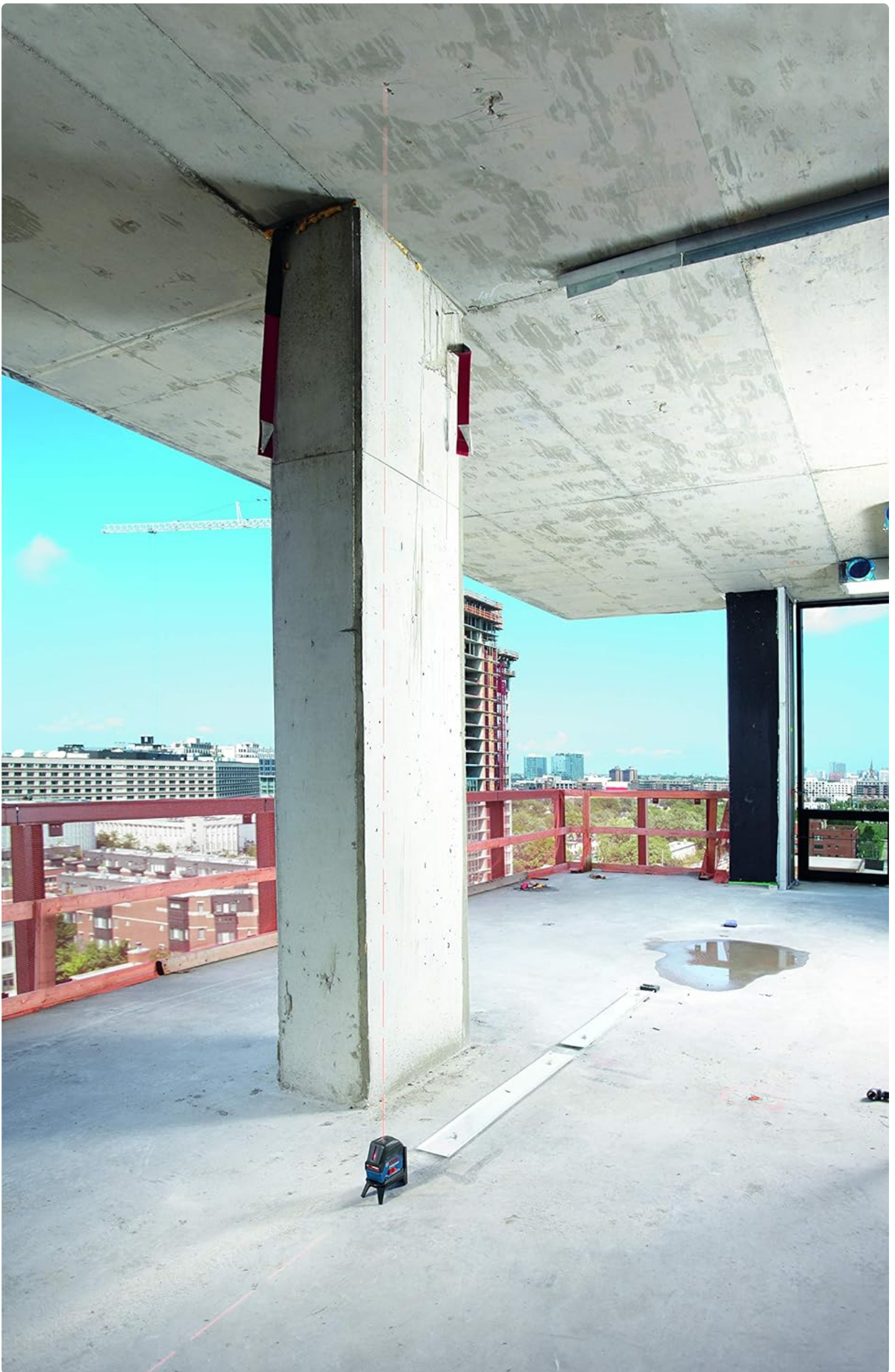
Figure 5: The Bosch GCL 2-160 boasts an accuracy of up to \pm 1/8 inch, a range of up to 165 ft (with receiver), and an IP54 rating for
