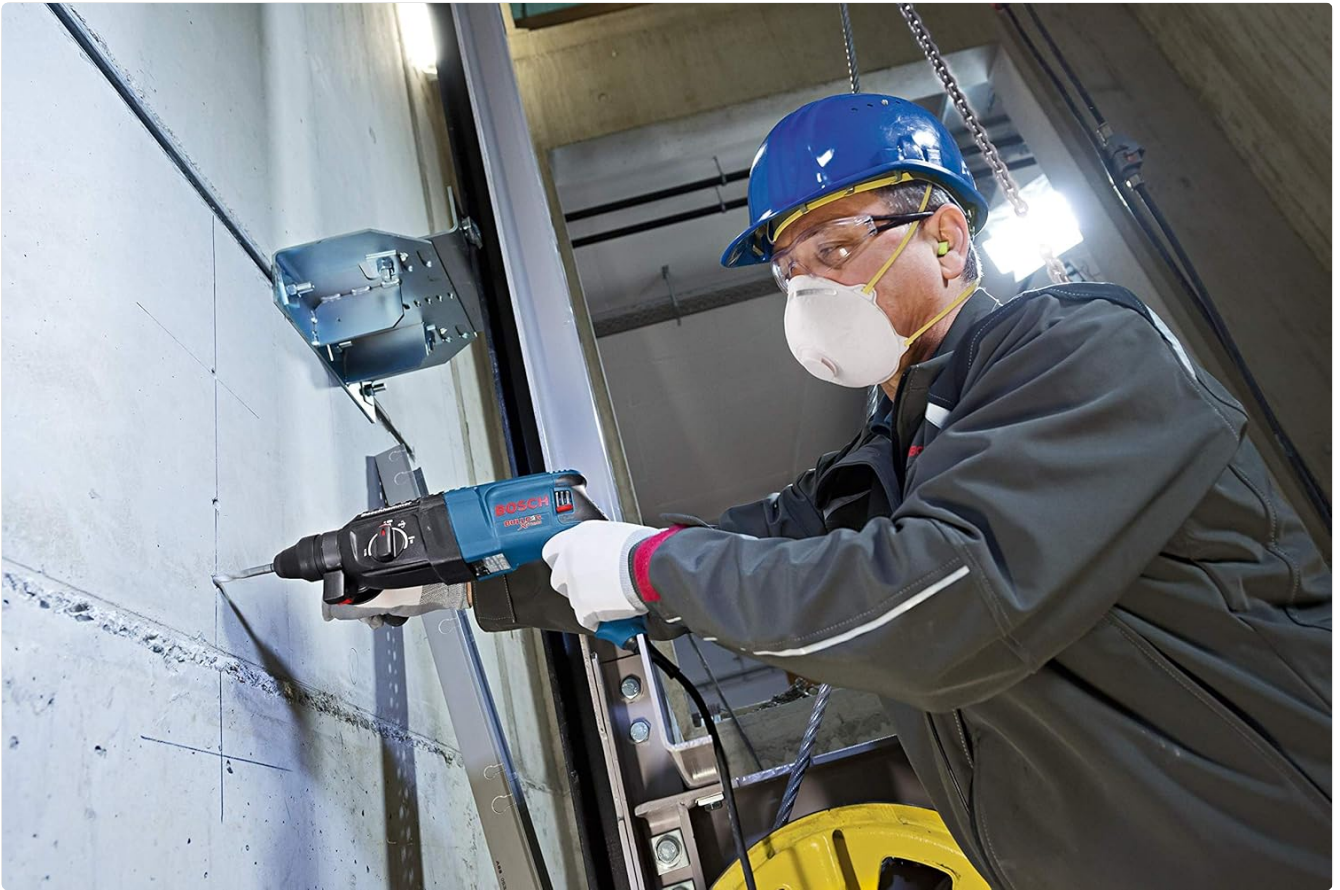
Figure 5.2: Drilling into a concrete wall using the hammer drilling mode.
