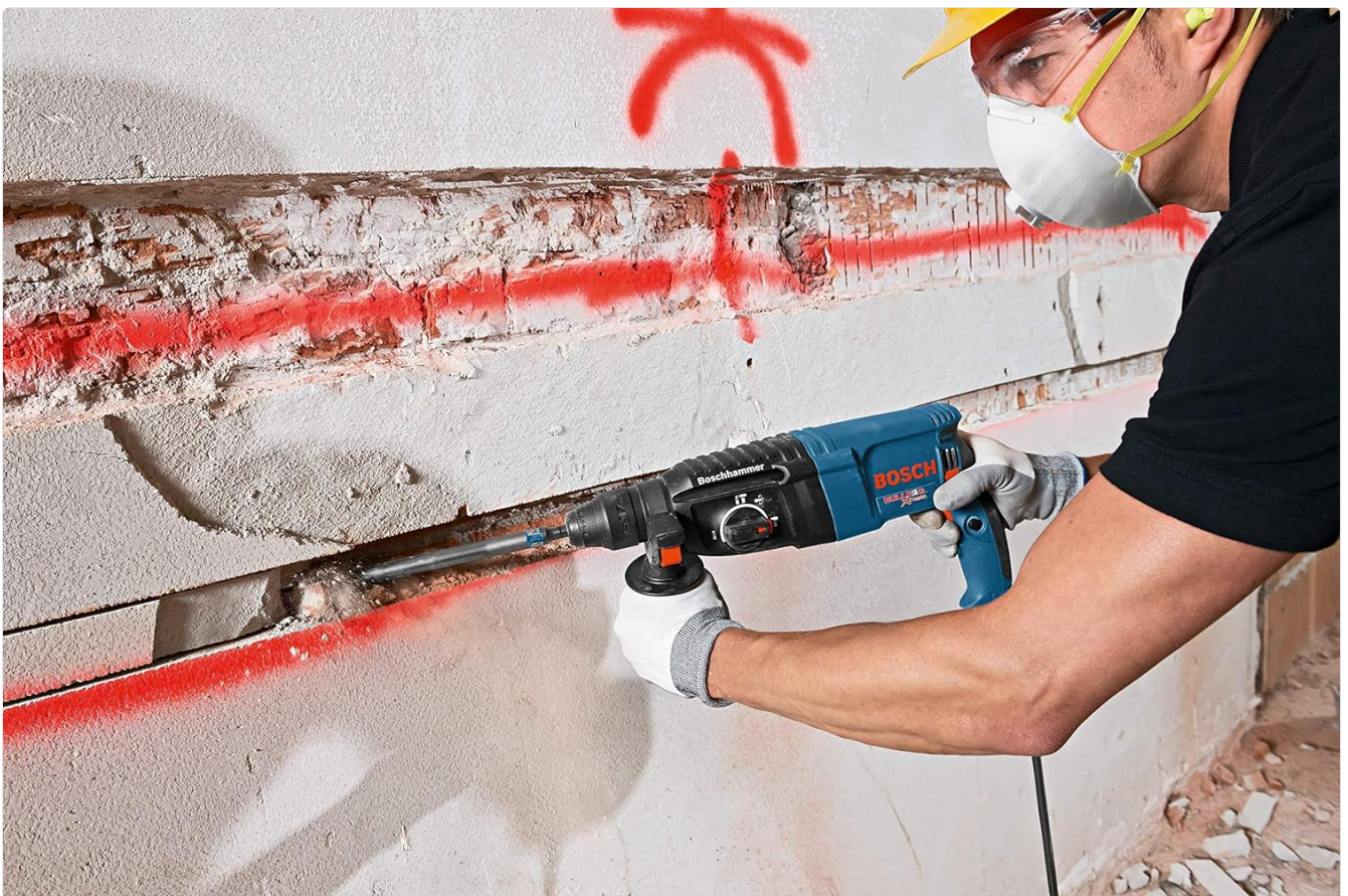
Figure 5.5: Chiseling concrete from a wall, showcasing demolition capabilities.
