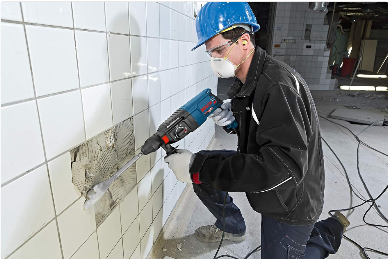
Figure 5.4: Chiseling tiles from a wall using the hammer only mode.
