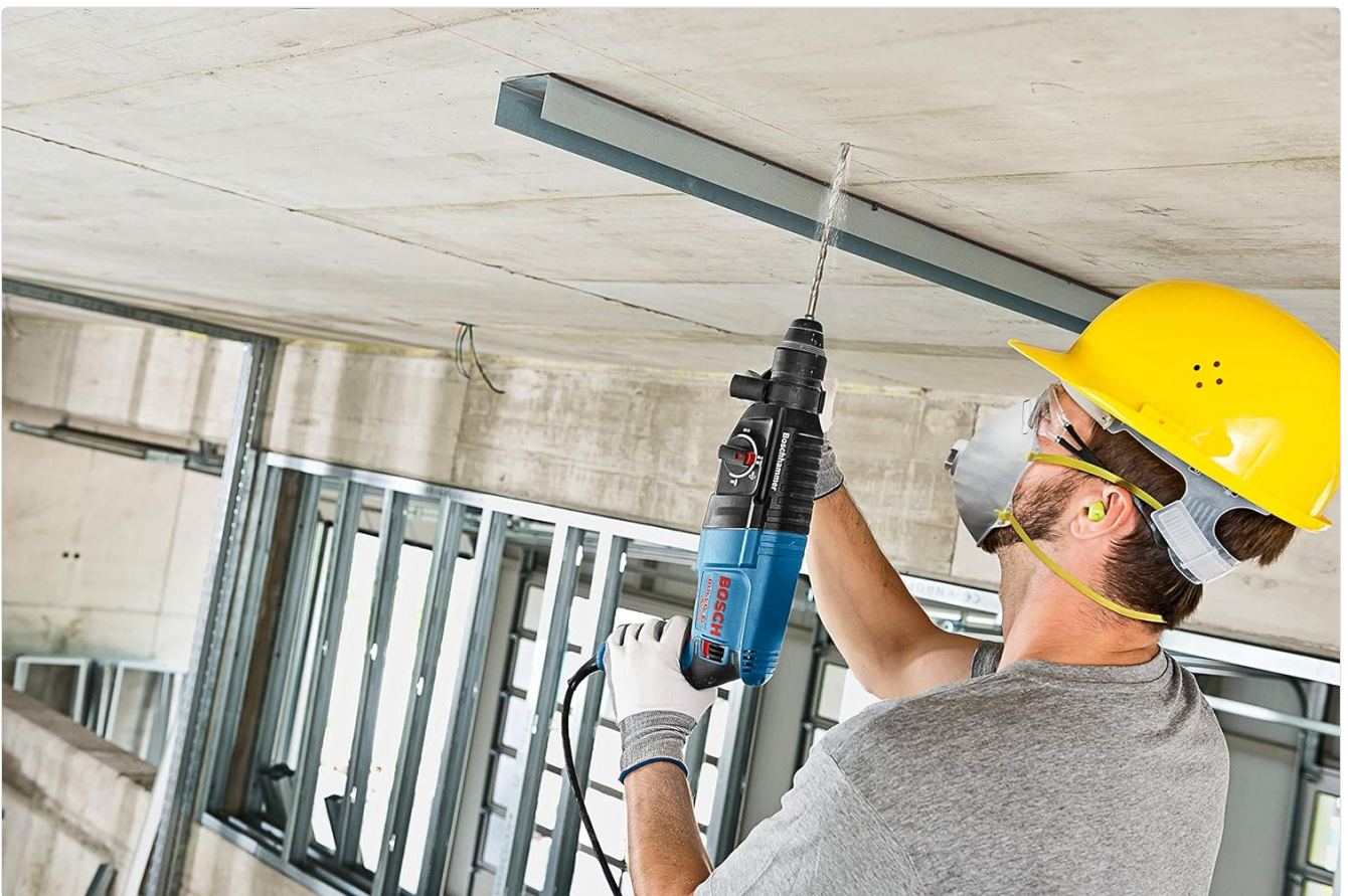
Figure 5.3: Drilling into a concrete ceiling, demonstrating overhead use.
