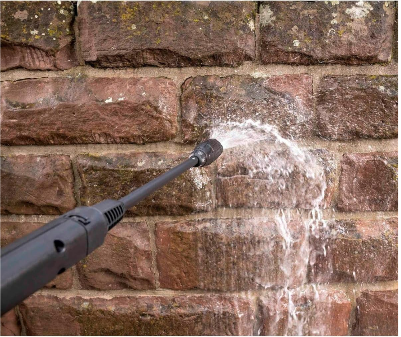
Image: High-pressure cleaning of a stone wall, demonstrating effective dirt removal.
