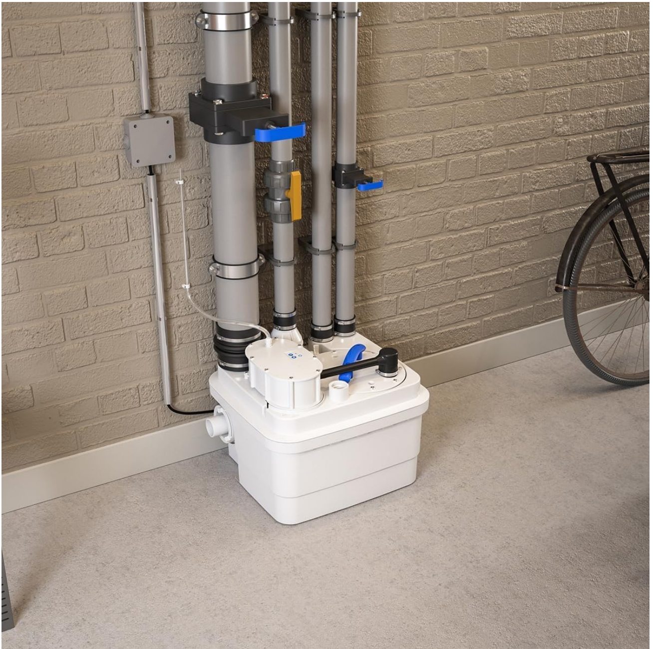
Figure 5.1: Example installation of the Sanicubic 1 in a utility room, connected to various plumbing lines.
