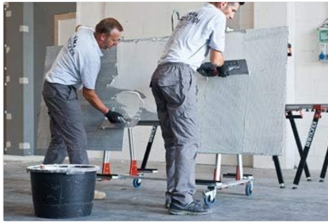
Figure 7: Two workers simultaneously back-buttering large tiles, demonstrating the efficiency of using multiple A Frame Carts.
