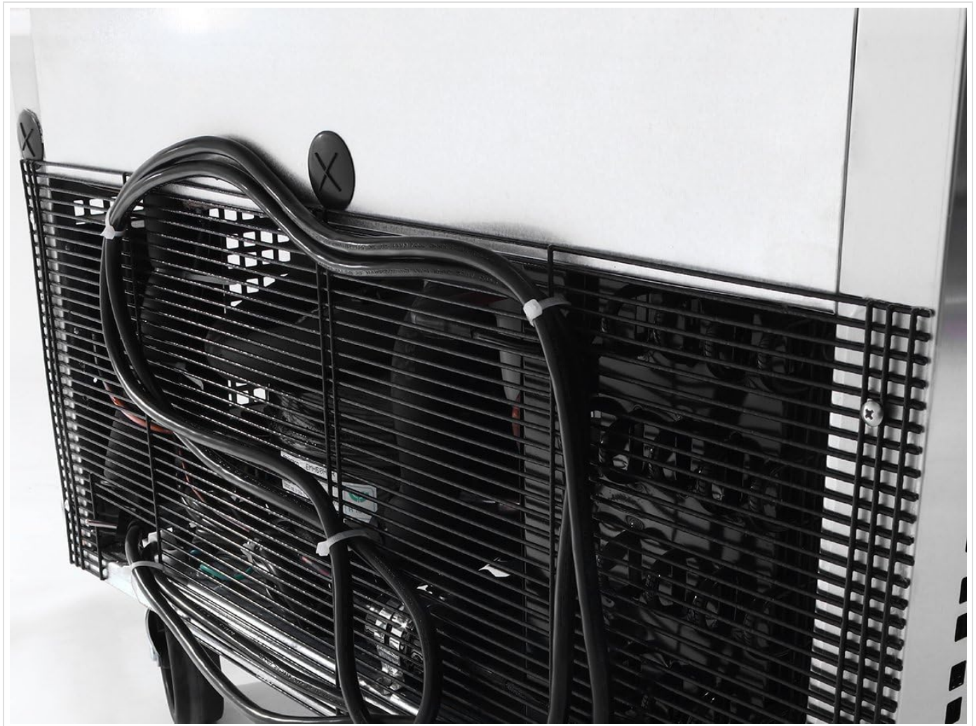
Image: The rear of the freezer, displaying the condenser coils and fan, which require regular cleaning for optimal performance.
