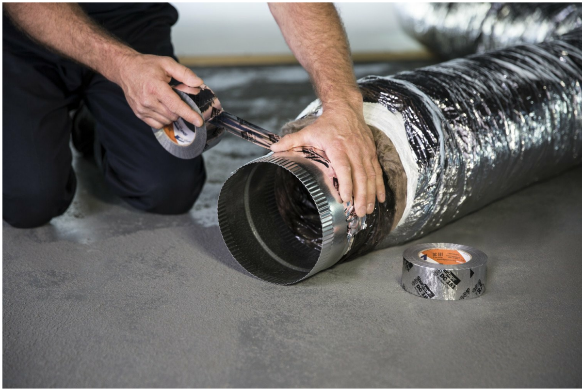
Image: A person applying Shurtape DC 181 tape to seal a connection on flexible insulated ductwork, demonstrating the application process.
