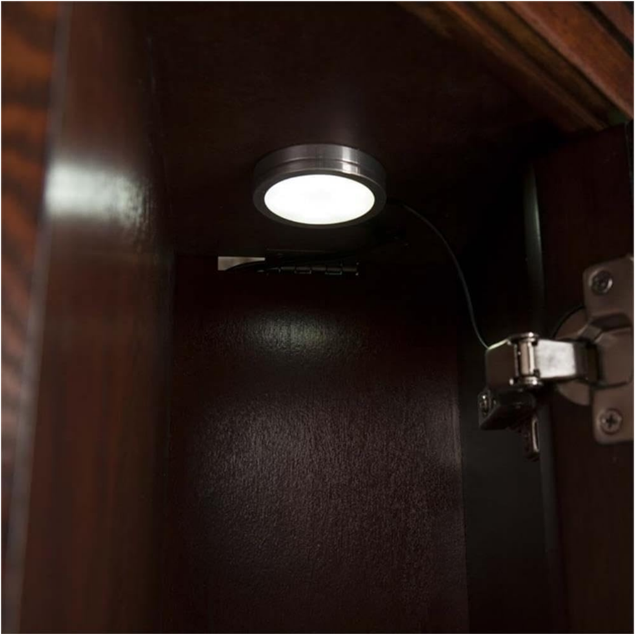
Image 7: A close-up shot of the circular LED light fixture installed inside one of the side cabinets.
