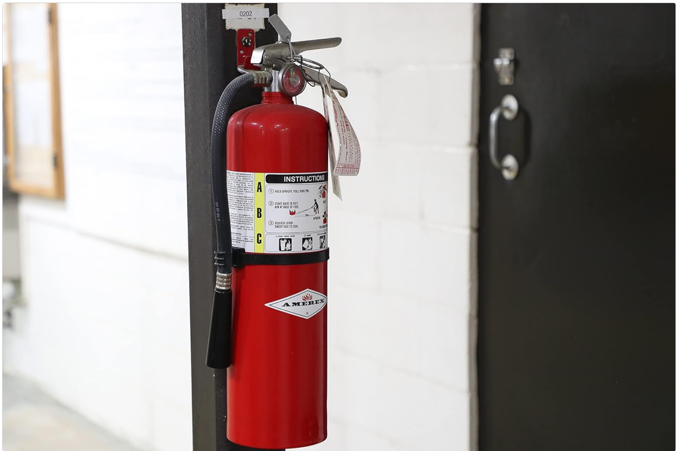
Figure 5: An Amerex fire extinguisher securely mounted on a wall using its included bracket, ready for use.
