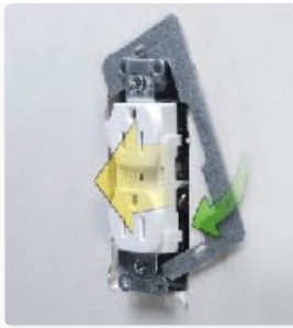
Figure 4: Illustration showing how to insert an electrical device, such as an outlet or switch, into the mud ring. Ensure proper alignment.
