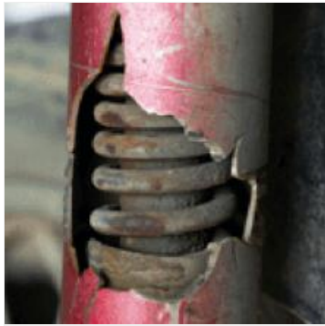
Image 5.1: Example of a corroded strut, indicating need for replacement.
