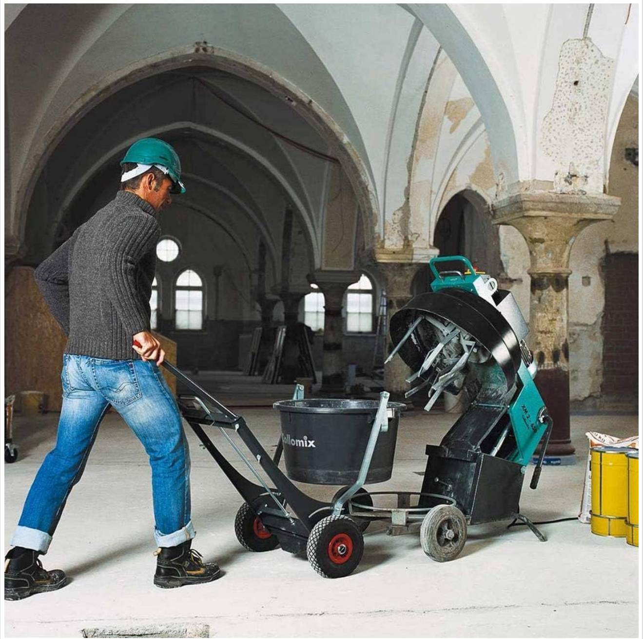
Figure 4.2: A worker operating the COLLOMIX XM 2 650 mixer, with the mixing bucket positioned on a bucket dolly. The dolly allows for easy movement of the mixer and its contents around the job site.
