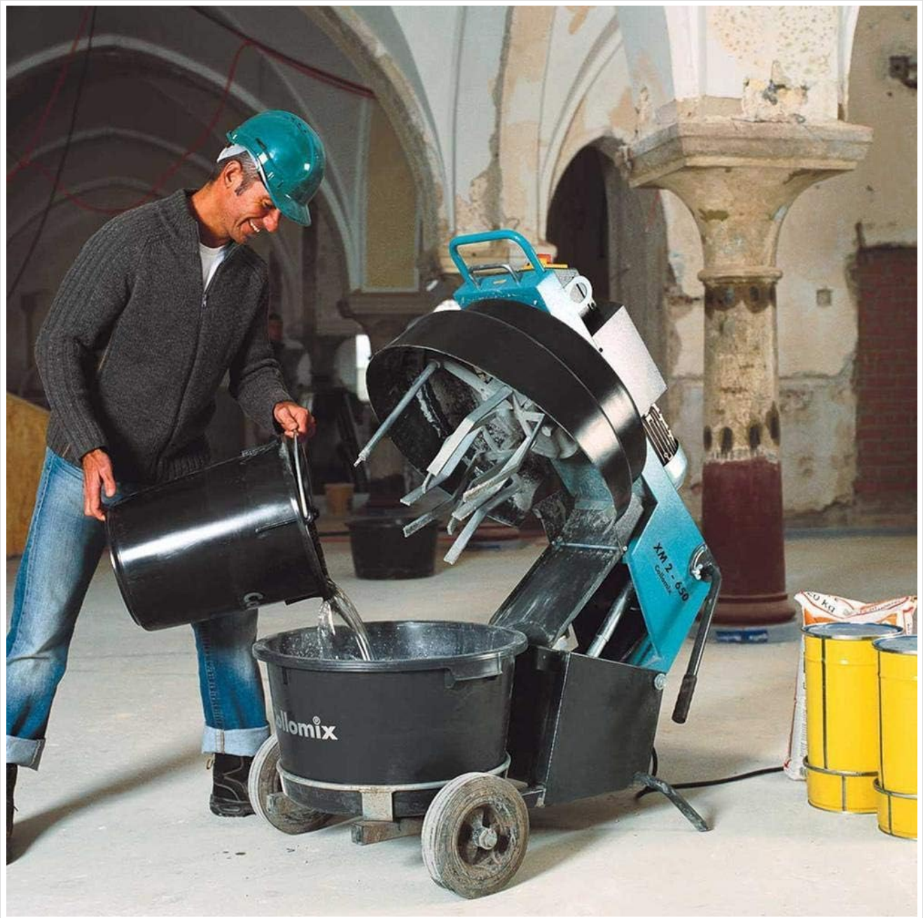
Figure 4.1: A worker carefully pouring dry material into the mixing bucket of the COLLOMIX XM 2 650 mixer. This demonstrates the loading process before mixing begins.
