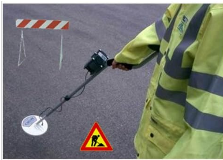
Figure 4.2: The CS880 in operation, highlighting its use in locating buried utilities on paved surfaces.
