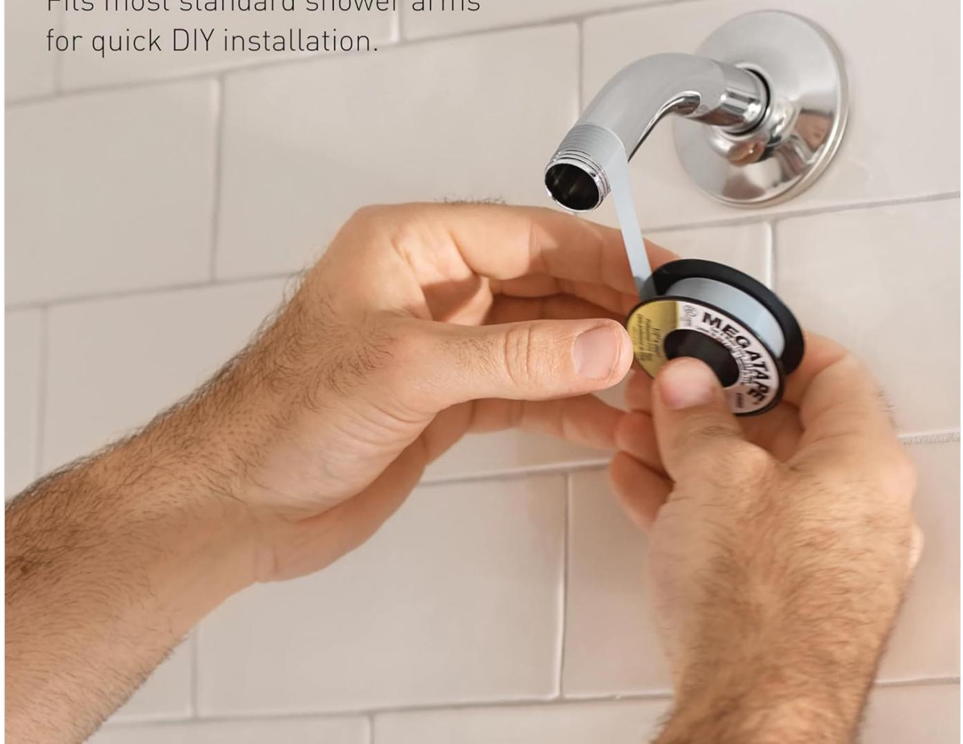
Applying plumber's tape to the shower arm is a crucial step for a leak-free installation.
