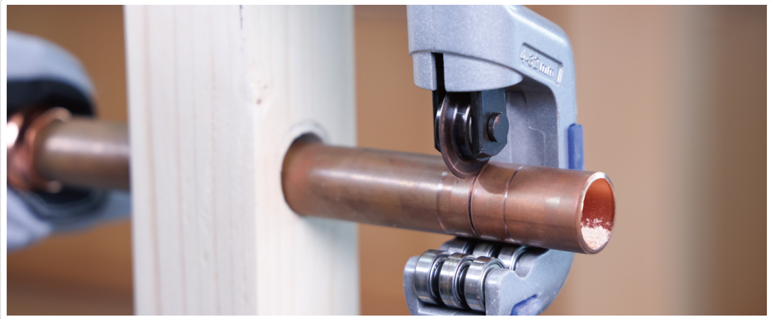
Figure 5: Cutting a copper pipe squarely for proper fitting.
