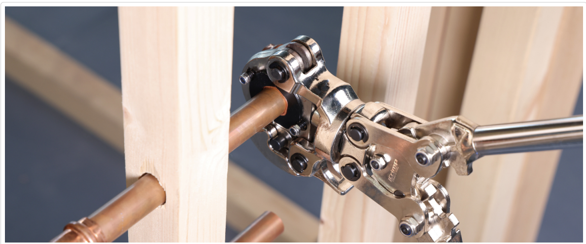
Figure 7: Positioning the crimping tool jaws around the copper fitting.
