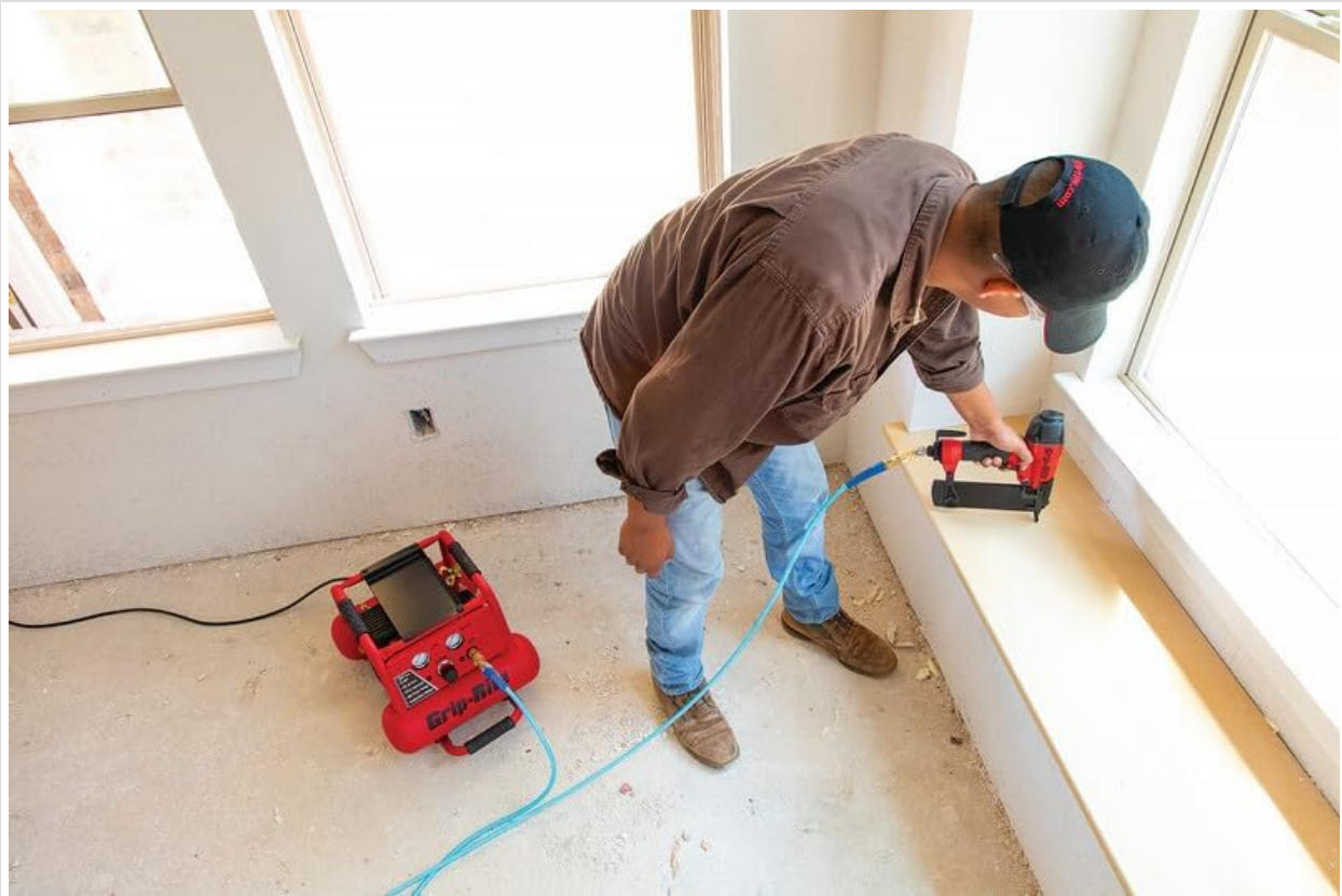
Image 4.1: A worker demonstrating the use of a finish nailer, connected to an air compressor, for fastening trim. Proper technique involves holding the nailer firmly against the material to ensure accurate nail placement.
