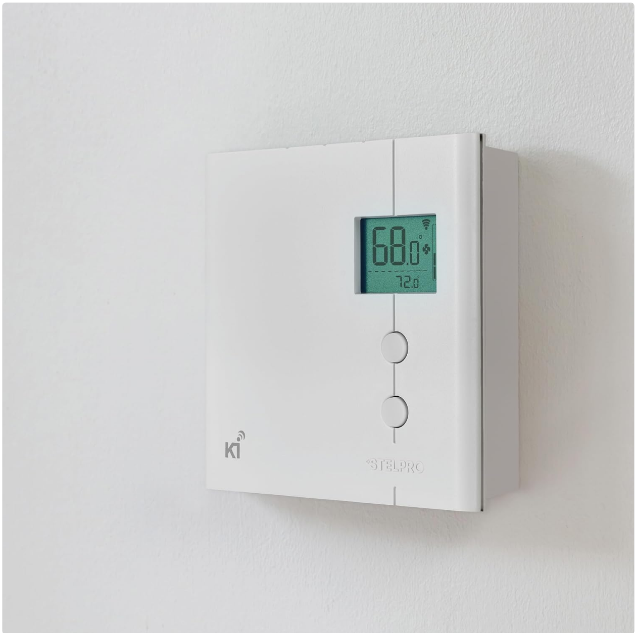
Figure 3: Stelpro KI STZW402WB+ Thermostat installed in a living space.
